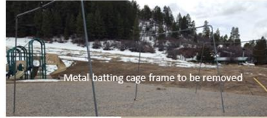
Existing Batting Cage Frame
